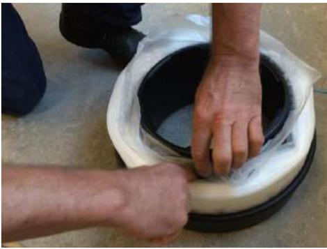
Pull the part of the bag that was put down into the centre of the dispenser over the rubber band
